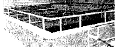
This Somersworth, N.H., Tricon™ plant treated river water to reduce color levels from an average of 100 color units to less than 5 color units, using only polymers as primary and secondary coagulants.
