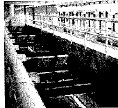
A 9.0 MGD Trident plant in Kokomo, Indiana, reduces iron and manganese levels.
